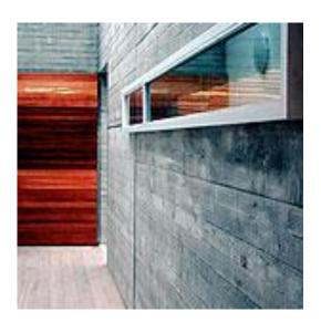
Constructed using 100mm shuttering boards, with careful alignment of openings and pour joints and control of cut out soffit surfaces it provides an exemplary concrete element contributing to a project of real quality.
