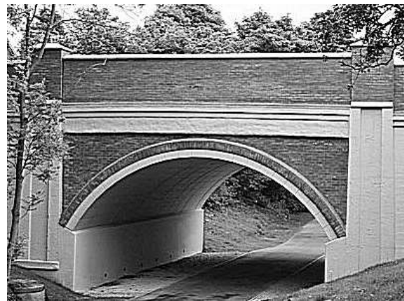
Figure 5. Ashton Bridge as restored (Construct Awards 2013)
