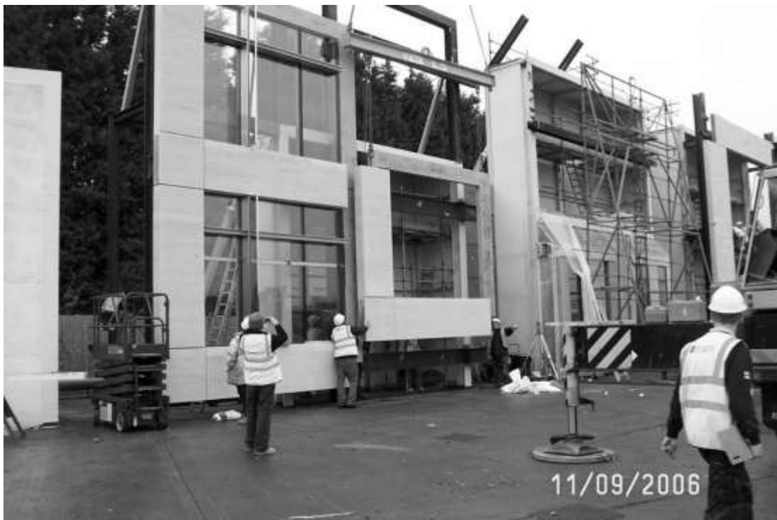
Figure 12. Ludgate Panel on Test Rig
