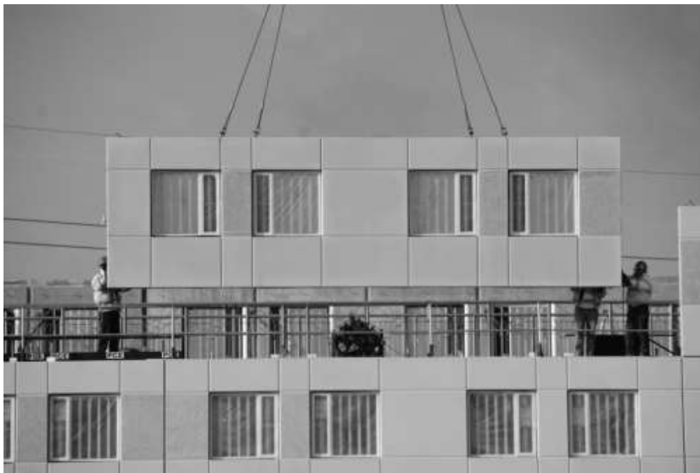
Figure 8. Featherstone Prison, panel being installed
