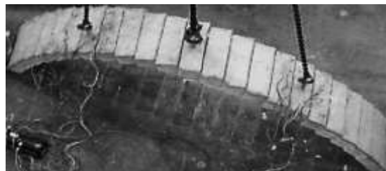
Figure 9. Lifting of skewed FlexiArch™ (McNulty et al, 2011)
