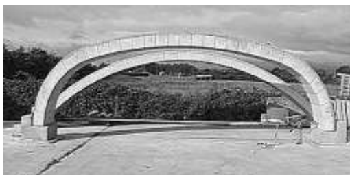
Figure 6. Double radius FlexiArch™ (Macrete 2012)
