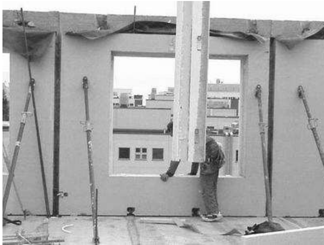
Figure 6. Internal view of load-bearing sandwich panels on site
