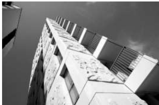
Figure 11. Use of CNC machine in mould formation for complex facade finish
