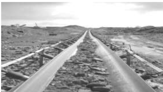
Figure 4(a) .Large capacity conveyor of c.1km length (B.D. Flood Ltd.)
