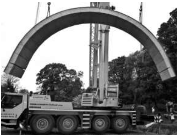
Figure 2. Lifting of FlexiArch TM (New Civil Engineer, 2008)
