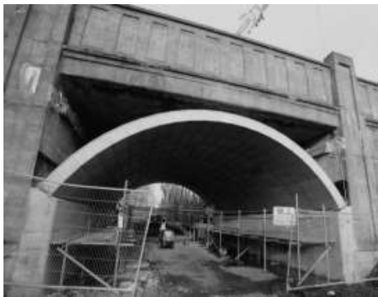
Figure 4. Insertion of FlexiArch™ (Construct Awards 2013)
