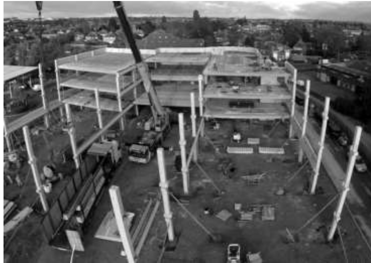
Figure 13. Multistorey Car Park During Construction
