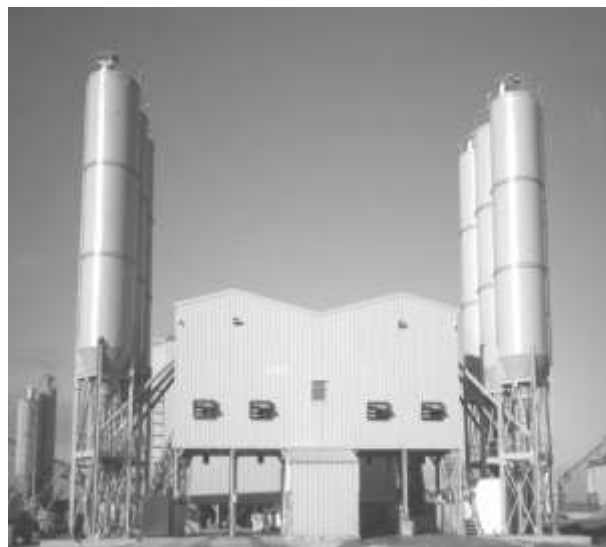
Figure 3 Modern twin wet batch plant
