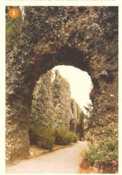
The Normans used sand and lime mortar in their buildings, and found that the addition of pounded tiles and bricks improved hardness and durability by producing a similar reaction to that of the Roman pozzolana.
