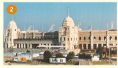
Between the World Wars, the use of reinforced concrete continued to expand. Wembley Stadium was built in 1923 in time for the FA Cup Final, when it is reputed to have held a crowd of 200,000. It is claimed to be the largest monumental building ever to have been constructed in reinforced concrete. At the time of writing it is not yet clear whether the famous twin towers will survive the extensive updating programme that is required to bring the stadium into the third millennium.
