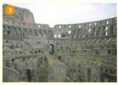
Lightweight concrete was used in some of the arches of the Colosseum, and also in the dome of the Pantheon, which is one of the few Roman buildings to survive intact. With a diameter of over 43 metres, its distinctive domed roof is a testimony to the durability of concrete, and was the largest dome in the world until the 20th Century. It probably inspired Sir Christopher Wren in his design for St Paul's Cathedral in London, the dome of which is only 34 metres in diameter.
