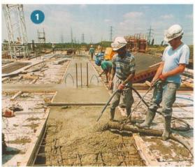
Concrete can be made on site, with the cement, water, sand and coarse aggregates being mixed either by using a concrete mixer or by shovel for very small quantities. Nowadays, however, most concrete is supplied to site by a ready-mixed concrete truck from a plant where it has been made accurately to precise specifications.
