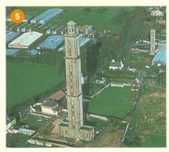
There are 11 rooms within the tower, which is surmounted by an octagonal observatory. The staircase is situated within an adjacent tower and comprises 330 precast concrete steps; the cornices and window mouldings are also precast.
