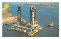
In the North Sea oil boom of the early 1970s, concrete was used to build some of the first production platforms and is still used today. These massive oil rigs are subject to harsh conditions where concrete's low maintenance needs and resistance to salt water come into their own.
