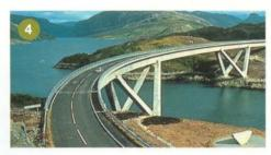
With modern techniques, spans approaching 300 metres can be achieved with the beam method of bridge construction. The bulk of our motorway bridges are constructed as beams, but generally have much shorter spans. They are a familiar sight throughout the country, forming intricate knots at complex multi-level junctions.
