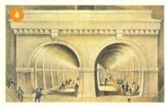
In his booklet, published several years later, William claims that Brunel carefully placed several tons of his cement into the river when the tunnel roof collapsed. This sealed the break and Brunel was able to pump the brick-built tunnel dry and then reline parts of it with mortar made with Portland cement. Despite the problems with its construction, this was the world's first significant underwater tunnel.
