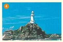
The first lighthouse to be constructed entirely from concrete was at La Corbière in Jersey. Built in 1873, it still stands on a very dangerous rocky outcrop to the south west of the island.
