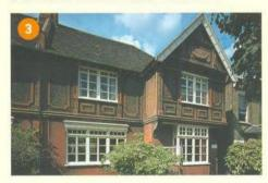
The houses consisted of a wooden frame to which panels, measuring about 1 by 0.75 metre and up to 40 mm thick, were fixed. The panels were usually made from crushed coke or cinders mixed with Portland cement. The mould was suitably prepared to produce an ornamental finish and in some cases iron oxide was added to provide a red colour. The red has since
