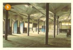
A wine and spirit store erected in Bridge Street, Reading, in about 1870 was another very large concrete structure. Built of mass concrete, it had four storeys. The walls were of solid concrete as were the floors, which were vaulted and supported on cast iron columns, each calculated to carry a load of 100 tonnes. After more than 100 years of service, the store was demolished to make room for new developments.
