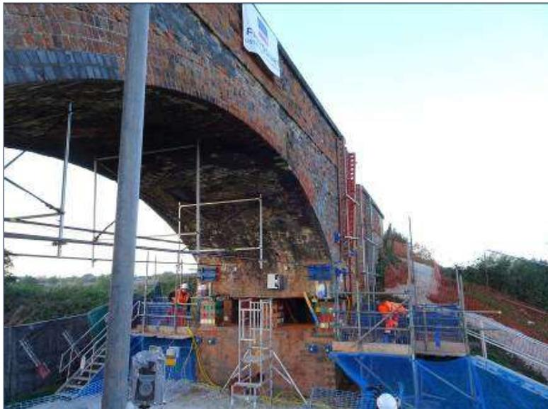
ElevArch® is a patented technique where the arch of a bridge is cut free from its abutments and walls so it can be jacked upwards, enlarging the space beneath. During the lecture, Bill will discuss the method and the technical difficulties of achieving such an innovative feat.
